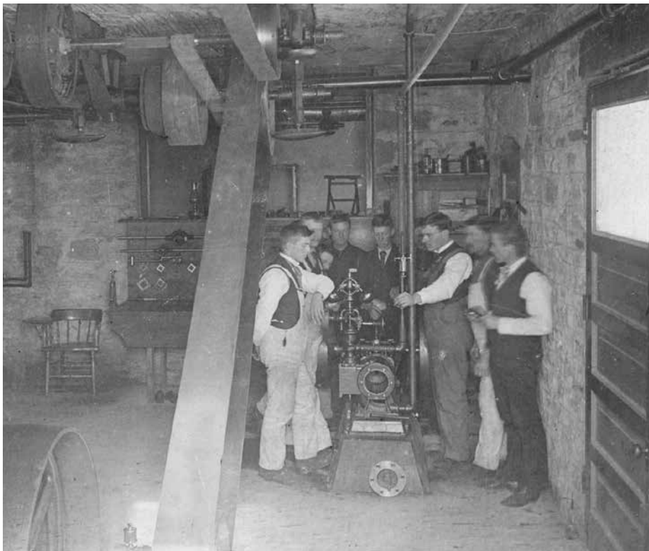
William Boss, right, in the trousers and vest to the right of the engine with his hand on the throttle, instructs creamery students in the initial class in steam engineering at the University of Minnesota’s dairy school. This photo from 1892 also shows how the power generated by the steam engine was transferred through a system of belts and pulleys to the creamery machinery on the floor above. Boss Family and Business Collection. Photo courtesy of the Minnesota Historical Society.
